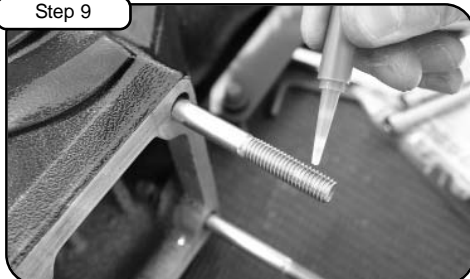
Step 9 Place threadlocker to all new manifold bolts.
