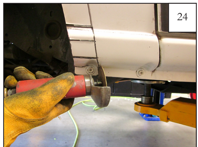
Using cut off wheel remove section containing bolt at the bottom pinch weld of fender. See step 25 for illustration of section to be removed.
