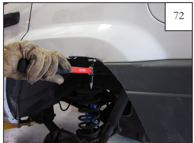
Use hammer to flatten tabs against inner wheel well.
