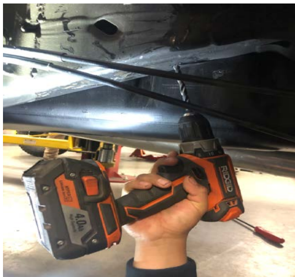
Figure 7: Drill Frame Mount Holes
