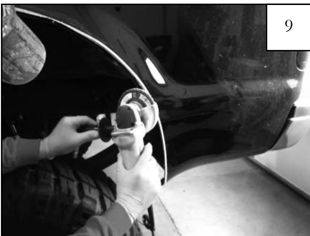
Using a grinder, deburr cut edges.
