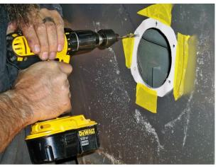
(Fig. 20) Cut out appropriate template and tape it around the 4.75" hole. Use center punch to mark screw positions and then using appropriate drill bit size, drill marked holes.
