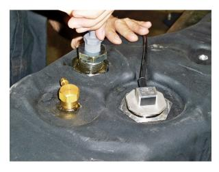
(Fig. 6) Installing ½" x 3/8" Hose Barb Elbow into plated Double Tapped Tank Bushing.
