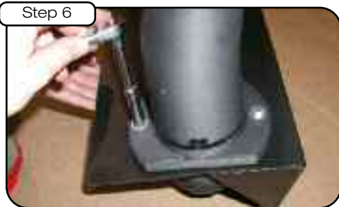
Insert tube into heat shield with flange on outside. The longer side of the tube should be facing outside of the heat shield. Secure using provided M6 hardware; be sure to use one washer for each side of each bolt, DON'T over-tighten.
