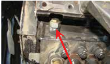
Figure 46 Return Line From the P-7100 Pump
